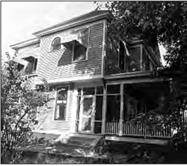
A sensitively designed second-story addition to the front side facade of this residence projects slightly beyond the screened porch over which it sits.
