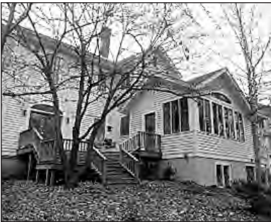
This contemporary rear addition with deck has been successfully differentiated from its principal structure, yet is compatible with the structure in design, materials, and details.
