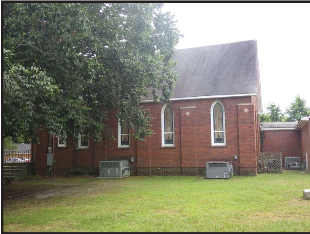
Figure 45. North Side Showing Buttresses with Concrete Caps
