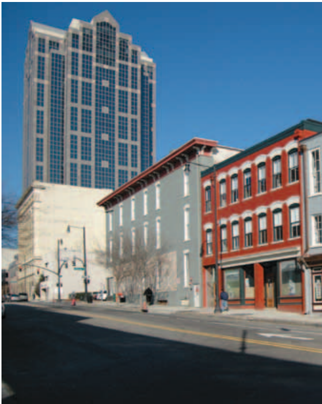
Many of the buildings along the Black Main Street in Raleigh have been rehabilitated, breathing new life and economic growth into this part of North Carolina’s capitol city. Courtesy of North Carolina Historic Preservation Office.
