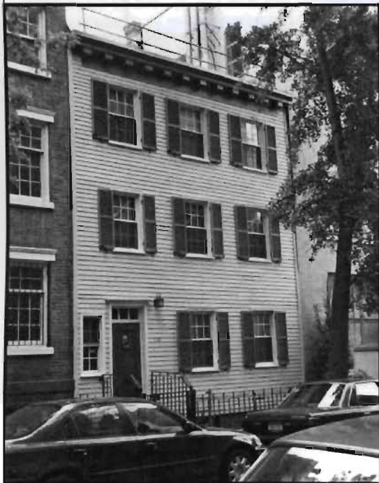
132 Charles Street in New York City is a rare example of a surviving wooden building. Photo: courtesy of the author
