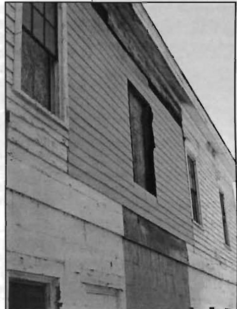
New fiber-cement siding on 1857 Merced Co. (California) courthouse. Photo courtesy of Mark Odell.
