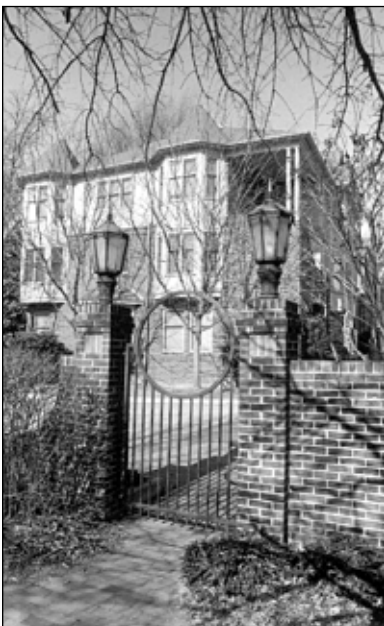
Sensitive siting and massing of the condominium complex at New Bern Place make this large-scale project compatible with the scale and the character of its historic context.
