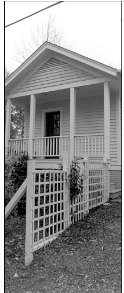
Site features should be considered an integral part of a project when planning additions to buildings.
