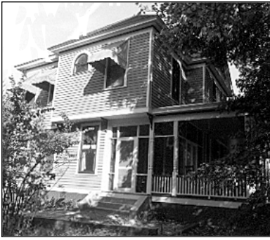
A sensitively designed second-story addition to the front side elevation of this residence projects slightly beyond the screened porch over which it sits.
