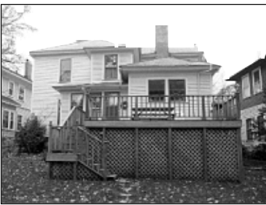
Wooden decks like these, located on rear elevations with simple balustrades, skirtboards, and lattice infill panels between supports, are appropriate in the historic districts.
