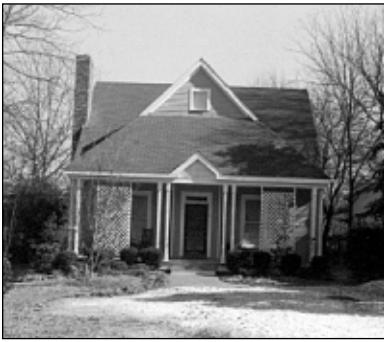
This new residence achieves compatibility with its Oakwood neighbors through similarities in height, mass, proportion, and materials.
