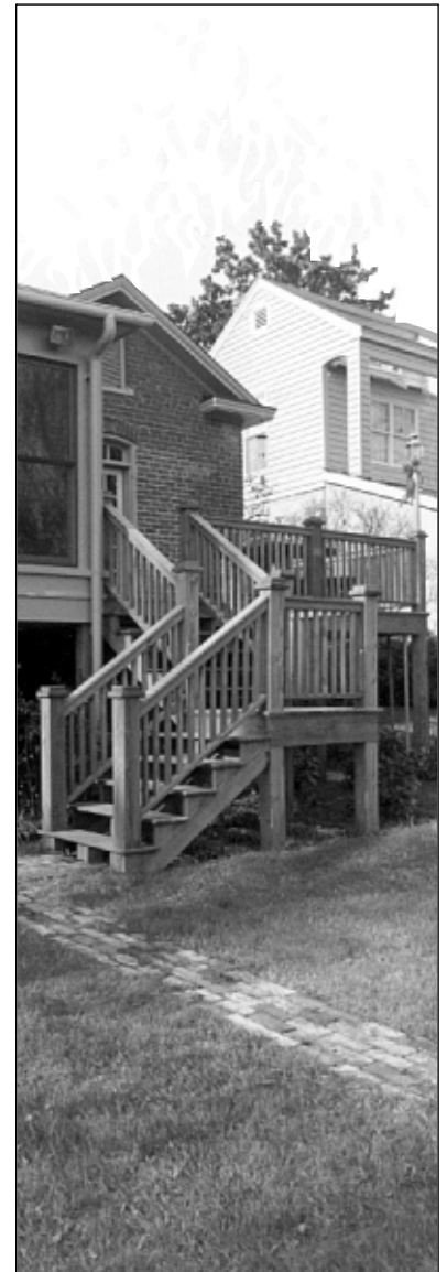
A carefully detailed deck stairway.
