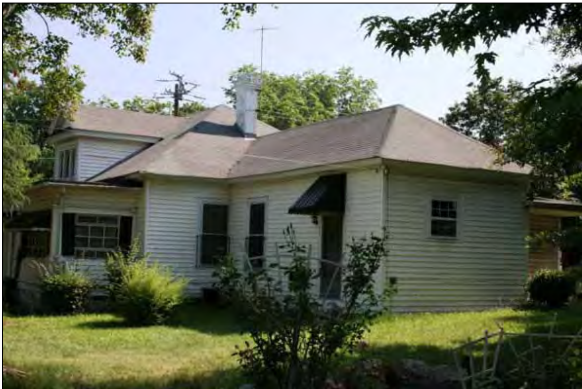
South Elevation (view from SW corner)
