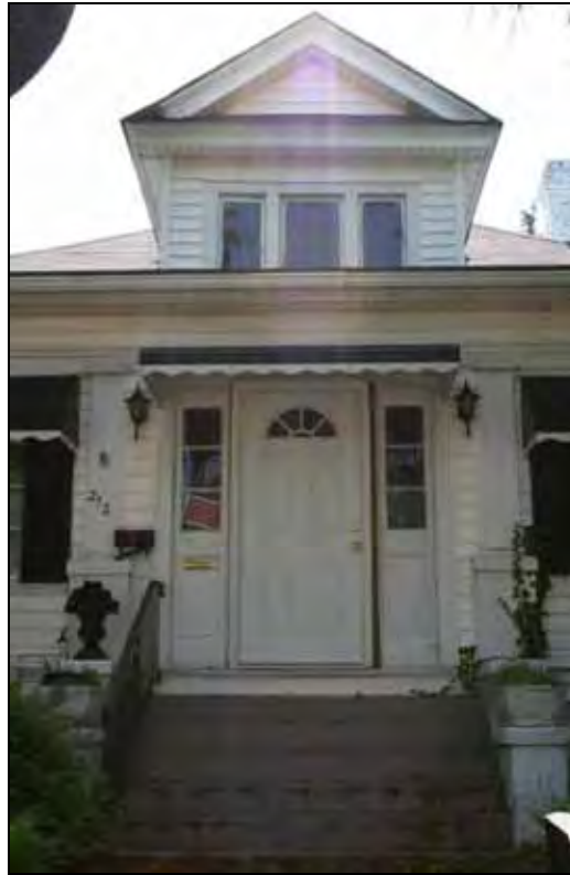
Front Door and Dormer Detail
