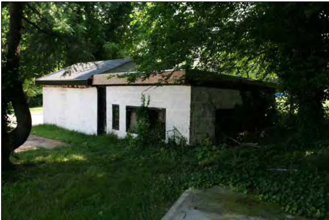
Garage (SW corner)
