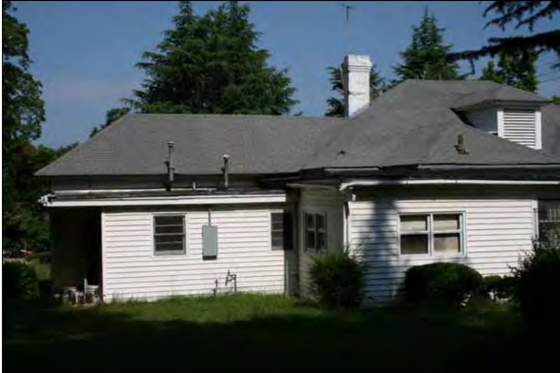
Rear/East Elevation (looking at rear of south wing)
