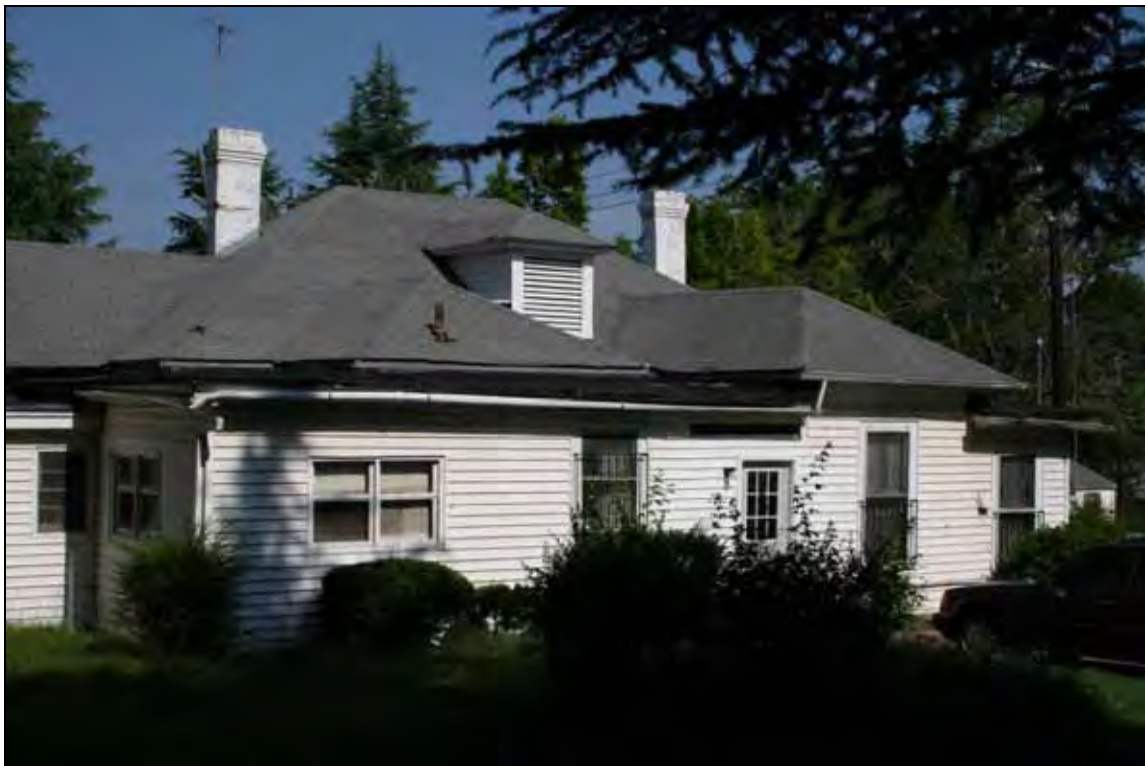
Rear/East Elevation (view of SE corner)
