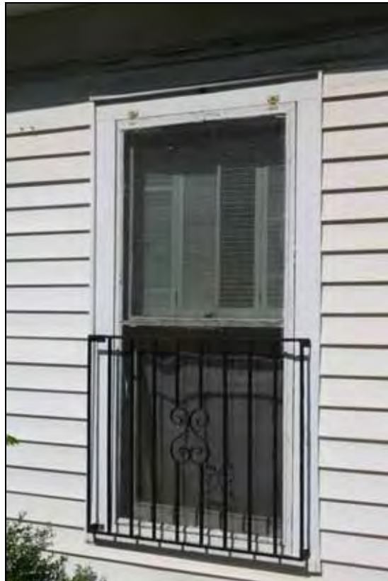
Original 1/1 Window with Screen (Rear Elevation)
