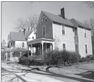
Formerly located on land acquired by Peace College for expansion, these residential structures now facing Person Street were successfully relocated instead of being demolished.
