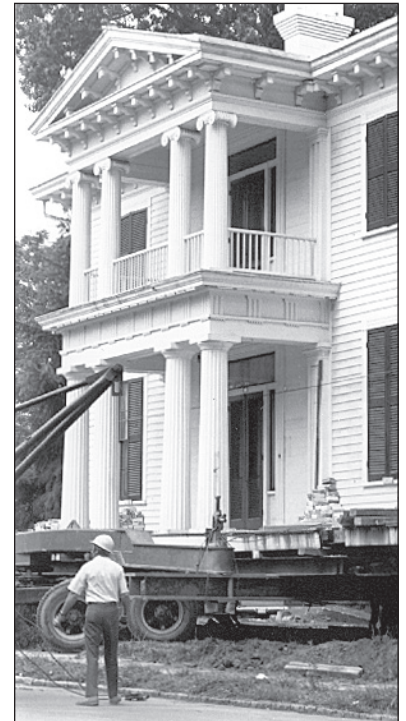
Even the two story portico of the Lewis-Smith House remained attached during its relocation.
