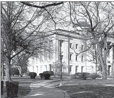
The Capitol Square Historic District centers on the State Capitol and its prominent square surrounded by churches and government buildings.
