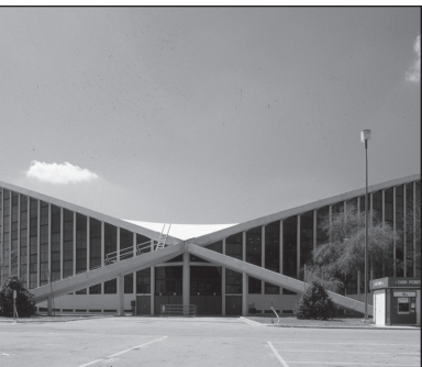
The J. S. Dorton Arena, built in 1952, a Raleigh Historic Landmark, is recognized for its exceptionally significant design that boldly combines architecture and engineering through its parabolic structure.
