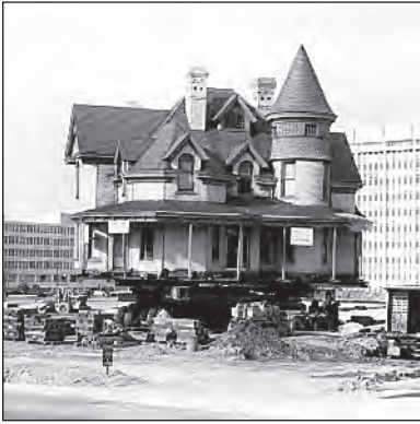
Both the Capehart House (above) and the Lewis-Smith House (below) were relocated within their neighborhood to Blount Street sites and were adapted to house government offices.
