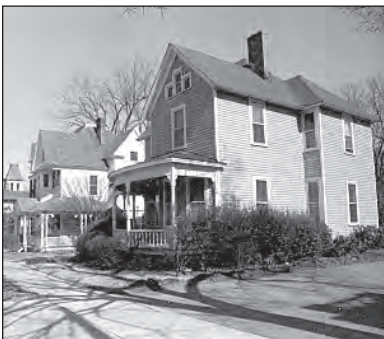
Formerly located on land acquired by Peace College for expansion, these residential structures now facing Person Street were successfully relocated instead of being demolished.
