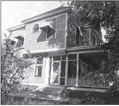
A sensitively designed second-story addition to the front side facade of this residence projects slightly beyond the screened porch over which it sits.
