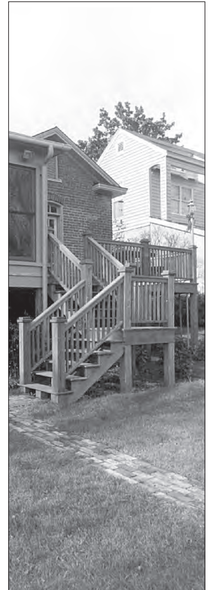
A traditionally detailed deck stairway.
