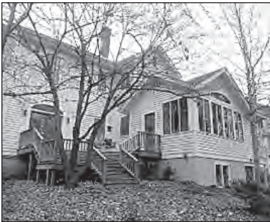
This contemporary rear addition with deck has been successfully differentiated from its principal structure, yet is compatible with the structure in design, materials, and details.
