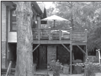
Tubular metal rods incorporated into the railings add contemporary detailing to this modestly-scaled wooden rear deck.
