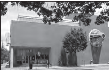
The side facade of this contemporary building also features a stepped wall clad in brick veneer, projecting corner sign, and a projecting glazed oculi.
