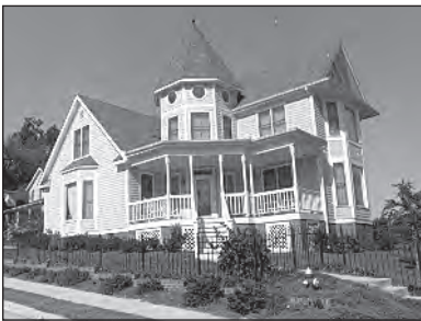
The compatible design of this new residence on a corner lot echoes the massing and the details of nearby Queen Anne-style structures.
