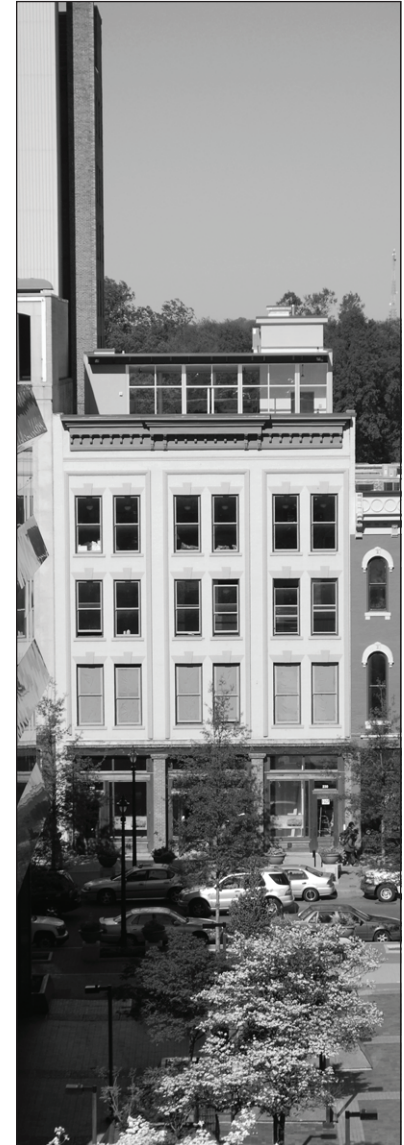
The rooftop addition to the Carolina Trust Building is setback so far from the Fayetteville Street facade that it cannot be seen from the street.
