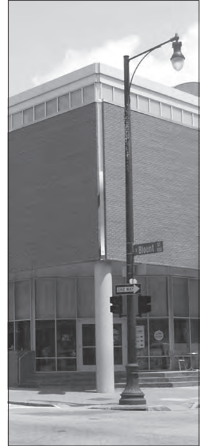
At street level, the corner of this building is recessed on the diagonal, yet a hefty concrete column establishes the building corner. Above it, the two brick veneer walls stop just short of meeting in the corner—another detail that differentiates this building from historic buildings in the downtown.
