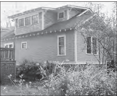
This upper floor attic addition echoes the design details of the original bungalow while respecting and retaining the original roof ridgeline and eaves.
