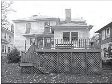
Wooden decks like these, located on rear facades with simple balustrades, skirt boards, and lattice infill panels between supports, are appropriate in the historic districts.
