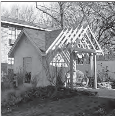
The design and the location of new garages and accessory structures in the districts echo those of their earlier counterparts; above, an accessory structure; opposite, a newly constructed single-bay garage.
