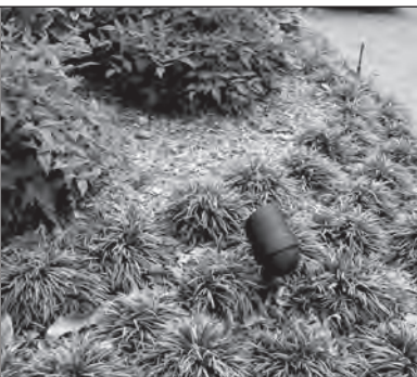
Site lighting in residential districts can often be increased unobtrusively and controlled through the introduction of carefully located directional lighting fixtures.
