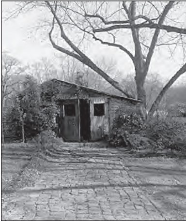
This early brick garage is sited in a traditional location near the rear property line at the end of a linear driveway constructed of granite pavers.
