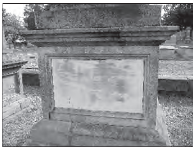
Unfortunately, the inscription on the marble face of this historic grave marker was damaged when it was cleaned with bleach and it is now illegible. Rather than falsify the stone by re-inscribing it, a new inscribed plaque could be placed nearby on a separate base.
