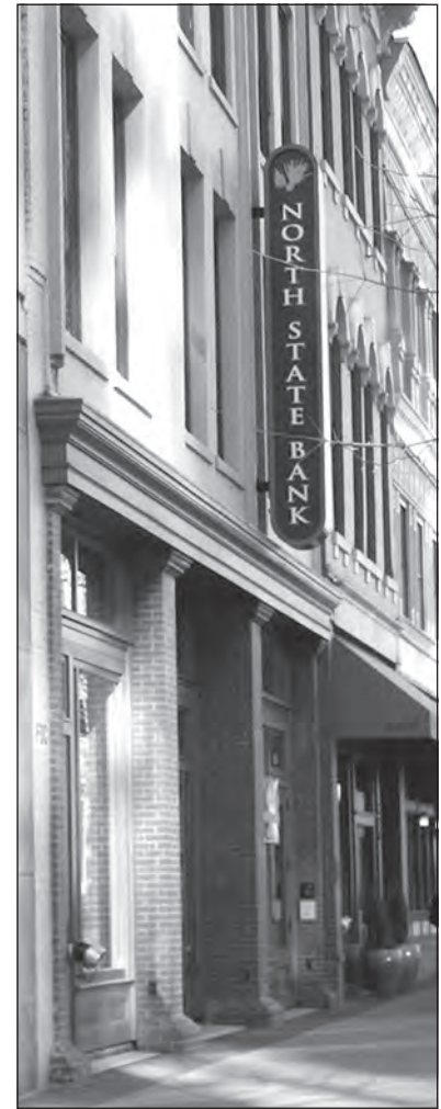
The new North State Bank sign above was constructed to match the original sign based upon historic photographs.
