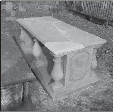
This tombstone was carefully pieced back together and a missing corner replaced by a skilled stone conservator.
