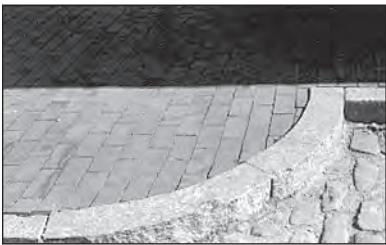
Retaining the granite curbing that edges so many district streets is important in preserving their historic character.
