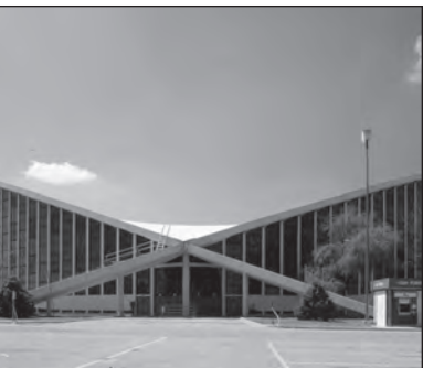
The J. S. Dorton Arena, built in 1952, a Raleigh Historic Landmark, is recognized for its exceptionally significant design that boldly combines architecture and engineering through its parabolic structure.
