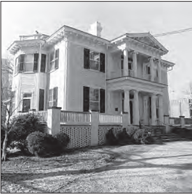
GREEK REVIVAL STYLE Lewis-Smith House, 515 North Blount Street
