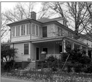
The second-floor sleeping porch on the side facade of this residence in Boylan Heights, though enclosed, retains its porch character.
