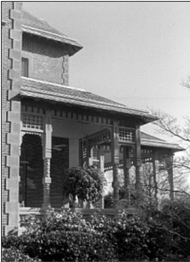
Ornate Eastlake-style porches and balconies wrap the facades of the Executive Mansion.
