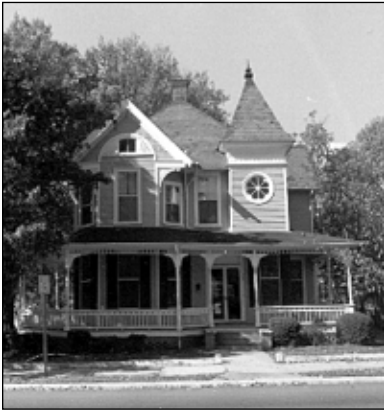
The projecting bay and tower of this asymmetrical facade are characteristic of Queen Anne-style architecture.
