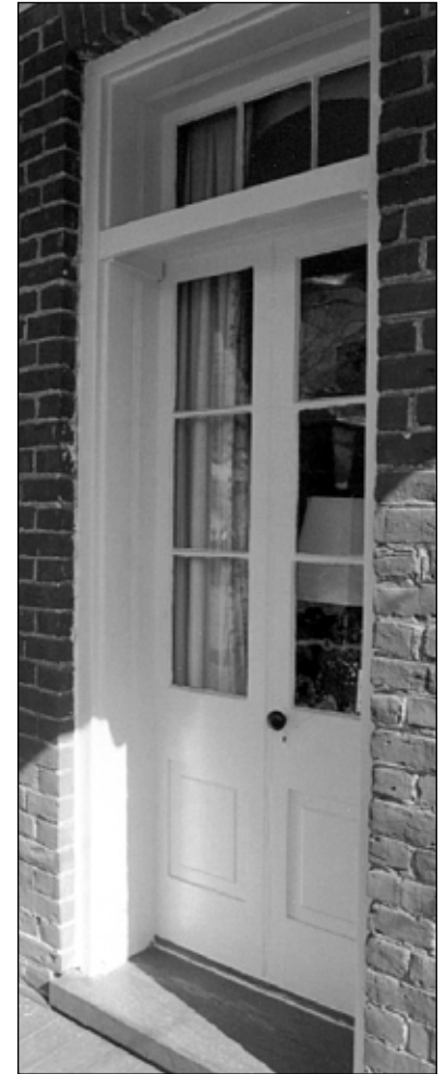
A distinctive entry with paired single-panel doors and transom above.
