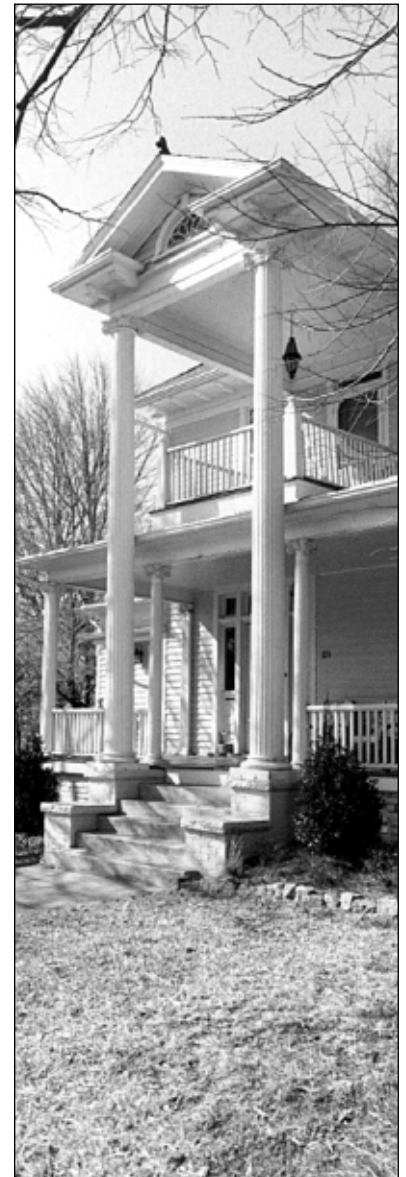
Porches are often a character-defining element for a building.
