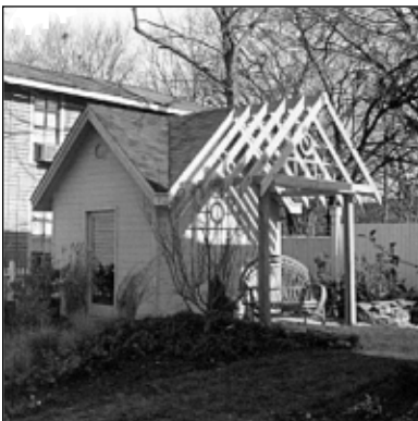
The design and the location of new garages and accessory structures in the districts echo those of their earlier counterparts; above, an accessory structure; opposite, a newly constructed single-bay garage.
