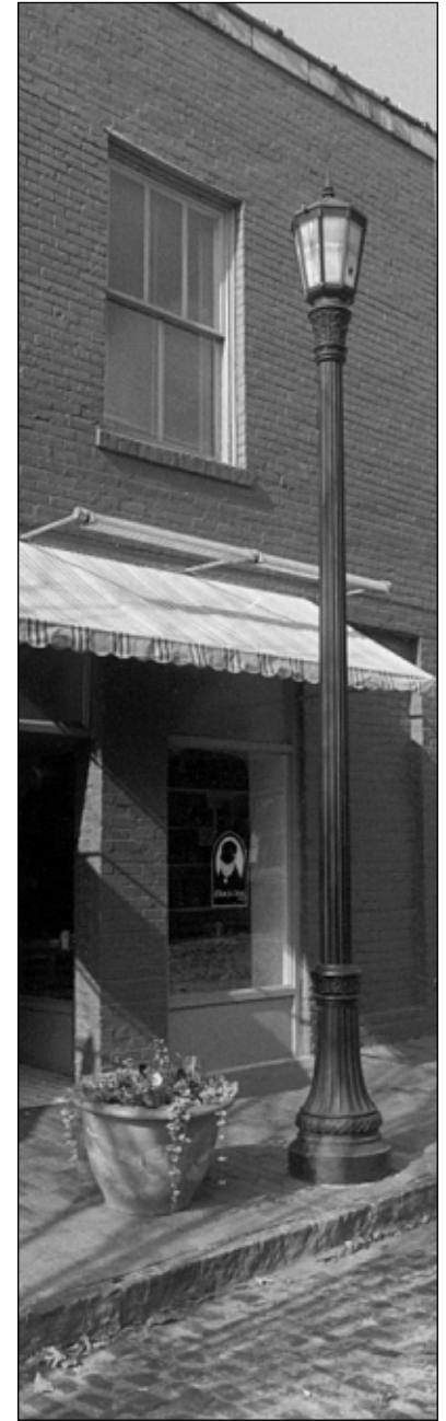
Compatible replacement streetlighting pole and fixture.
