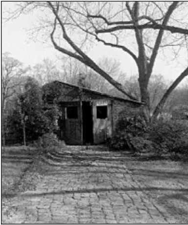
This early brick garage is sited in a traditional location near the rear property line at the end of a linear driveway constructed of granite pavers.
